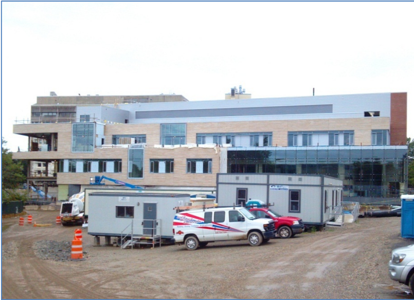
Figure 3 - New Academic Classroom Building
