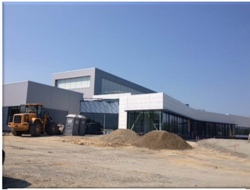
Figure 10 : MAB - Exterior Construction
