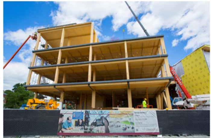
Design Building Being Built with Wood Structural Systems
